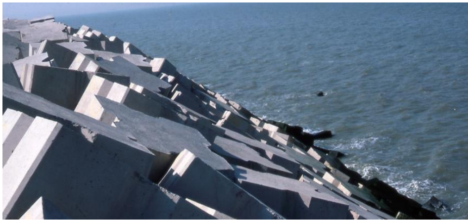
Figure 10 Antifer Cubes in the Port of Zeebrugge.
