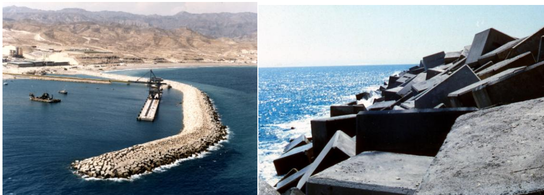
Figure 9 Puerto de Carboneras Breakwater. Cross section in deep water and photos of the port and armour layer.
