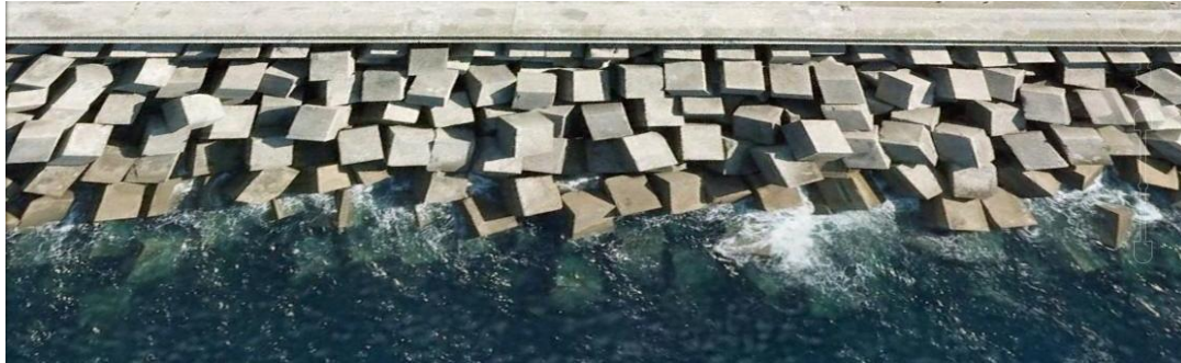
Figure 8 The armour layer on the Bilbao Breakwater 2013 (Google Earth).
